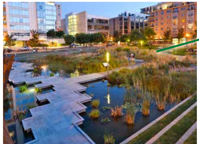
Tanner Springs Stormwater Park in Portland, OR Image via CMS Collaborative : a Vision Image of what sort of park could be integrated here
