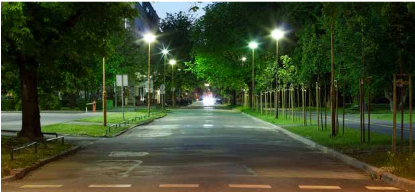
LED lighting is more illuminating and has become less expensive for street lighting improvements. Image via brandonindustries.com
