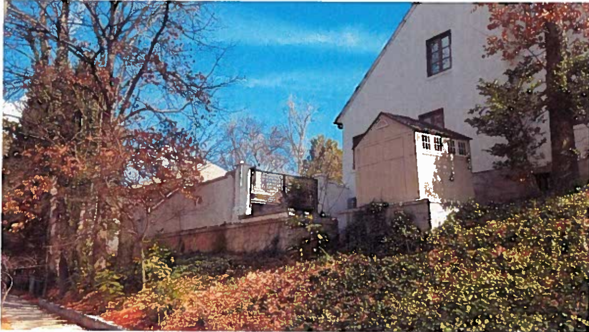
LOOKING AT WEST SIDE OF HOUSE/YARD, EXISTING SOLID BRICK FENCE
