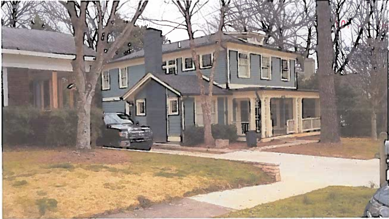
Adjacent two-story home (south side of property)
