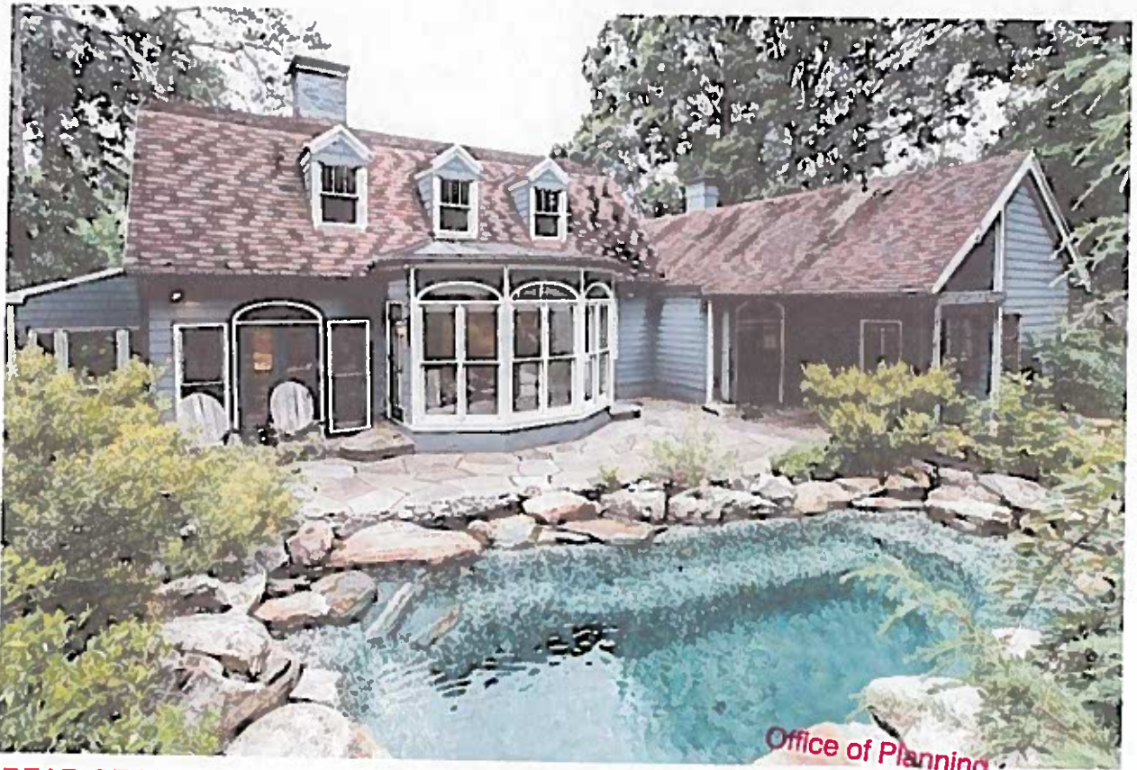
REAR OF MAIN STRUCTURE: LOOKING EAST POOL, MATURE LANDSCAPING, PATIO
