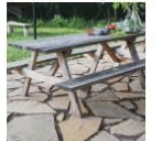
8. PERMEABLE FLAGSTONE PAVING IN PICNIC TABLE AREA
