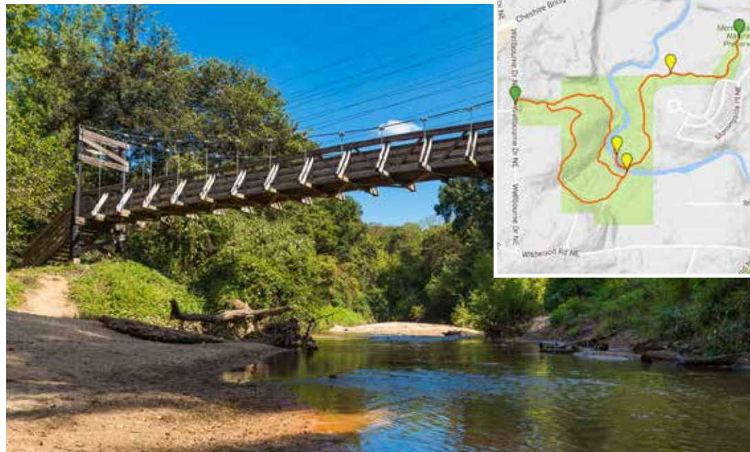
Famous suspension bridge in the Morningside Nature Preserve Image via atlantatrails.com
