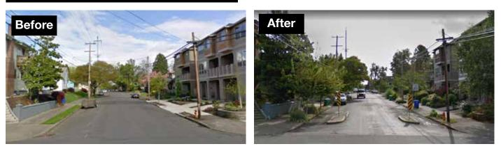
One-Lane Slow Points can further be installed with a raised crosswalk or speed table and depending on the width of the Slow Point mechanism, can also integrate landscaping elements.
