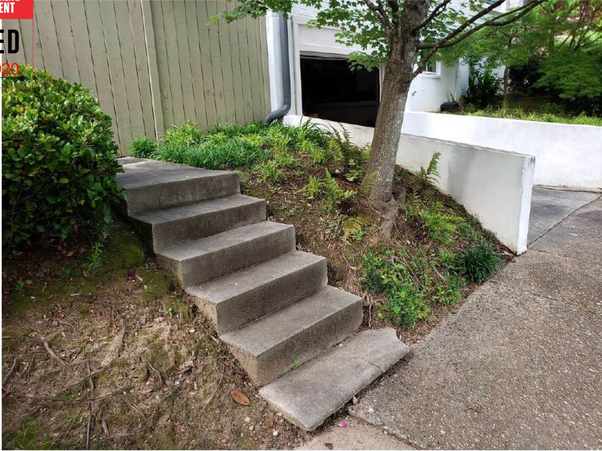
Existing concrete stairs to be removed
