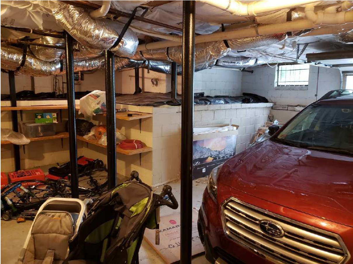
Tight conditions in existing small garage
