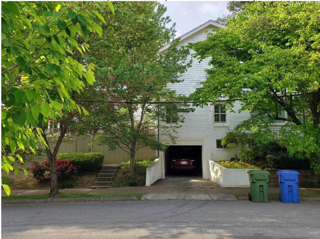
Side facing Courtenay Drive with two small trees (left of existing garage door) to be removed
