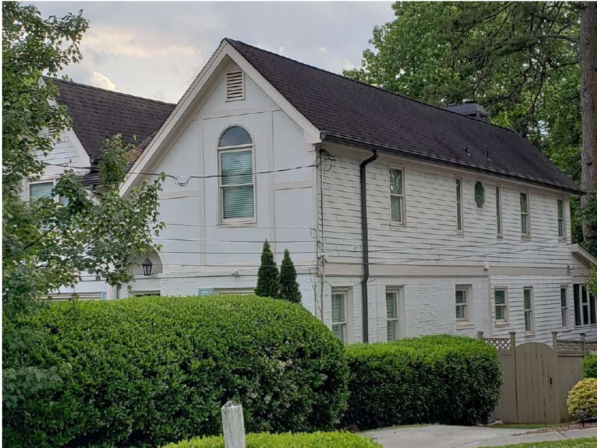
Right (north) side of house – no work on this side.
