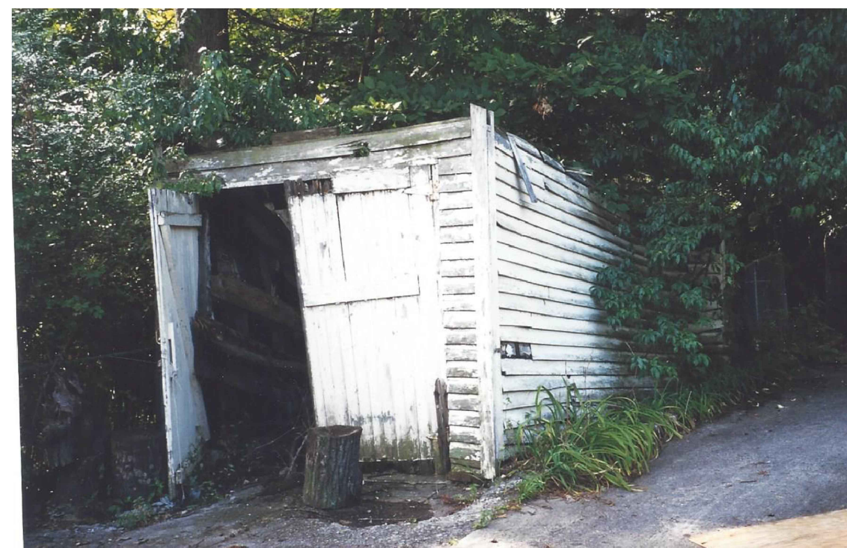
5 Photo of previous garage on location A2.01 NTS
