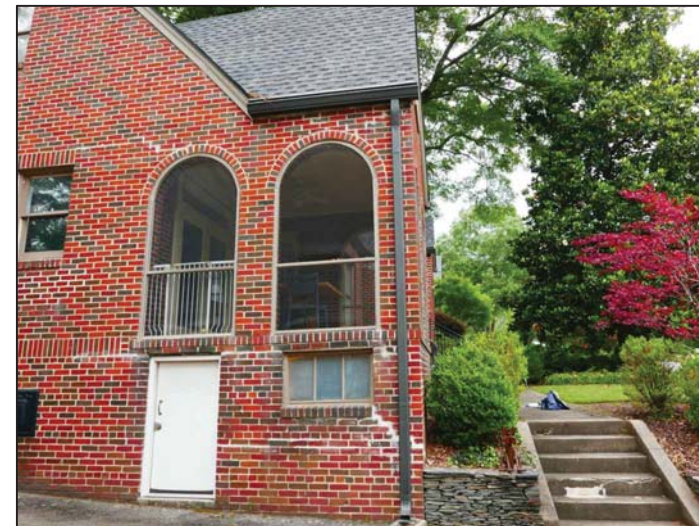
EXIST. SIDE OF FRONT HOUSE
